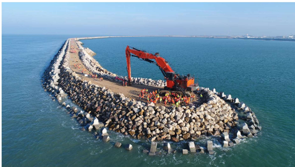
Figure 3-2: Breakwater construction at the Port of Calais
