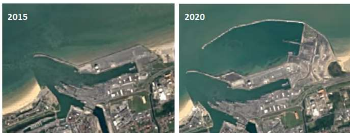
Figure 3-3: Port of Calais development status in 2015 and 2020
