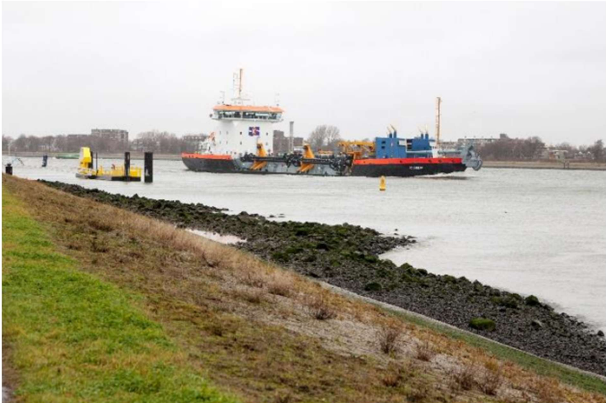
Figure 4-3: Hydraulic dredger Ecodelta at the reallocation site
