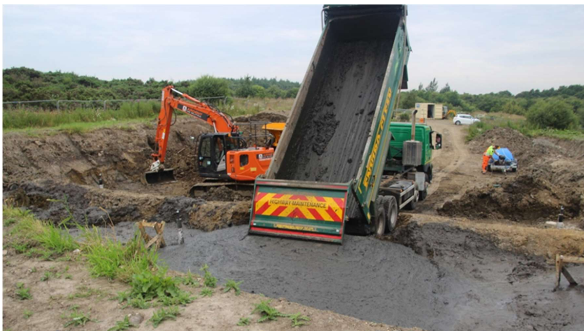
Figure 5-2: Falkirk site - dredged sediment placement
