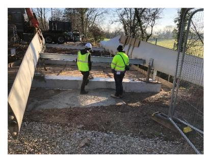
**Figure 9.** BladeBridge during assembly showing the cradles supporting the blades (prior to installing all the deck beams and plates).
