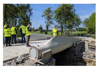
Figure 10. BladeBridge following installation on the Midleton to Youghal Greenway.
